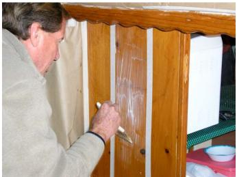
Figure 6-2. Brushing Stripper on Panel
